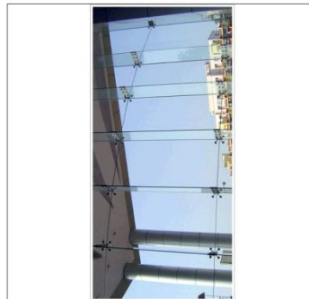
GLAZING glass fin system with spider fixings toughened glass with transparent finish.
